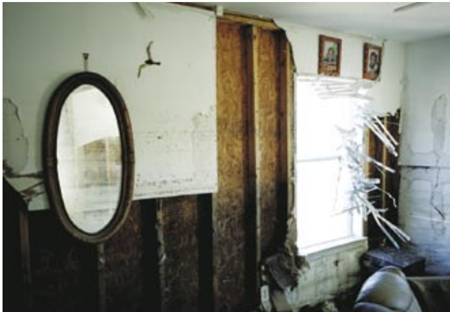
KATRINA STRIPPED the walls to the studs and smashed the window blinds on the first floor of a year-old home in the New Desire development. A mirror that survived reflects further damage.
